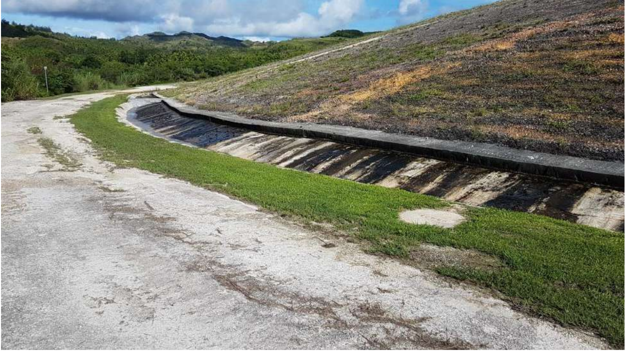
1. East PLCT MH-9 cover looking in a southwesterly direction.
